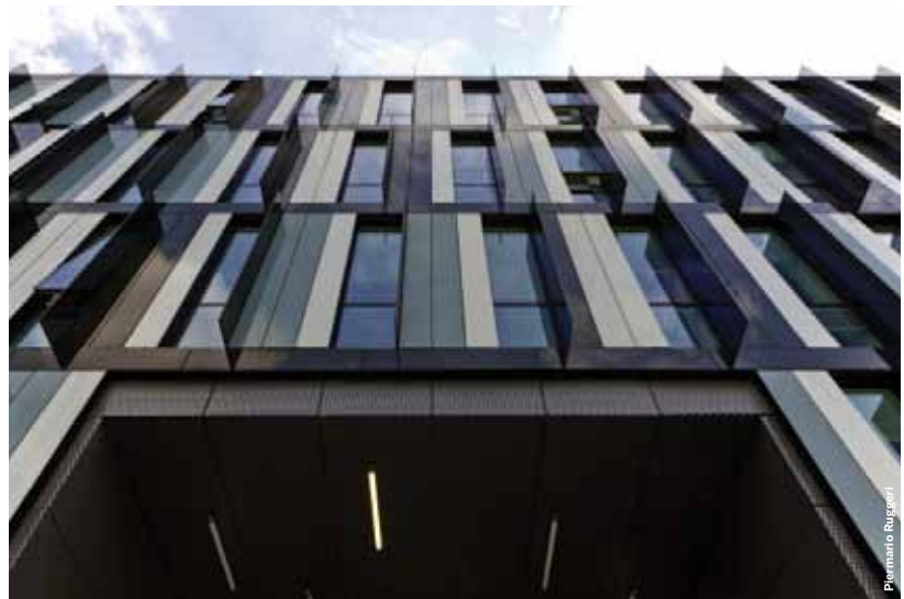
✓ RCS Headquarters B5, Milano - Barreca & La Varra Architetti (Focchi Spa)
